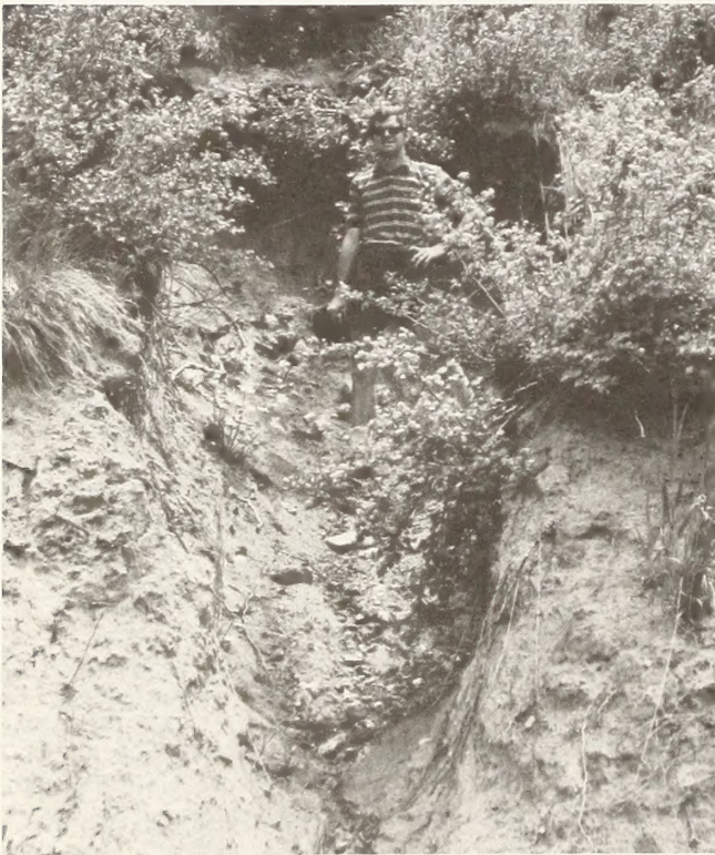
Figure 11. — Large gully in slope, Watershed No. 1, Pine Creek study area, Boise National Forest, Idaho. Gully was formed by subsurface flow emerging at cut face followed by piping and "spring sapping," which triggered localized slope failure. (Photo taken July 1977.)
